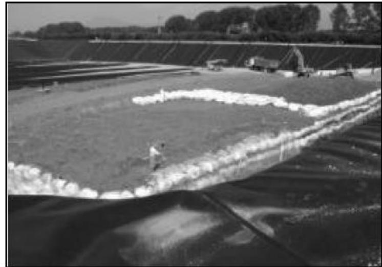
Fig 1. Disposal of asbestos containing waste at the dedicated cell of the Barricalla landfill.
